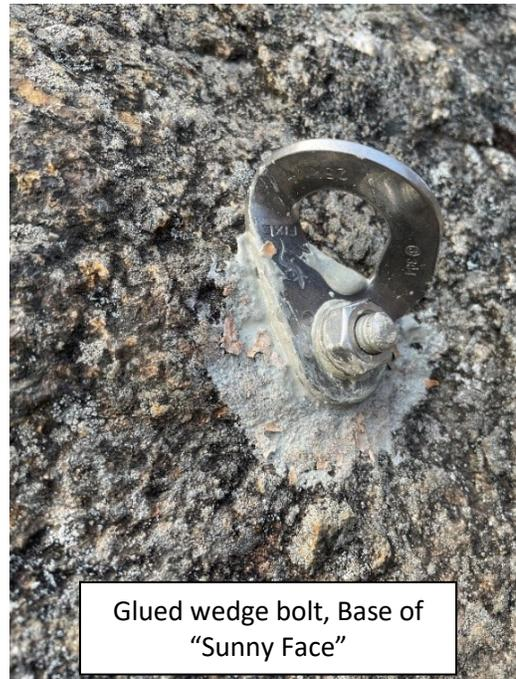
Glued wedge bolt, Base of “Sunny Face”
